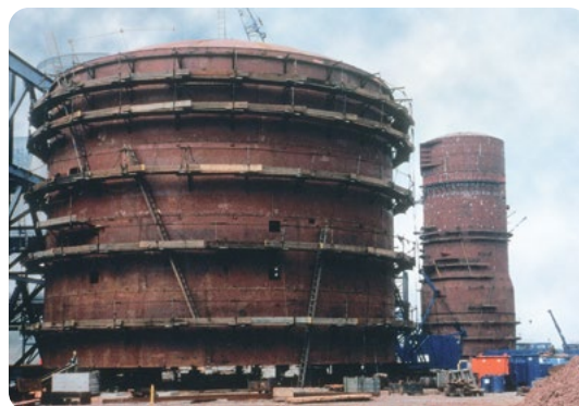
One Split-Flow ® pump can supply multiple jacks for accurate synchronized lifting without flow dividers.
